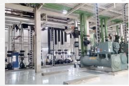
Removal of ozone depleting liquids from HVAC plants
